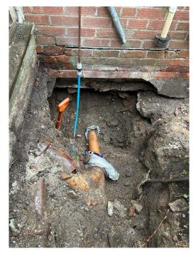
Subsidence damage (brown arrow) to the brickwork above the leaking drain (red arrow).
